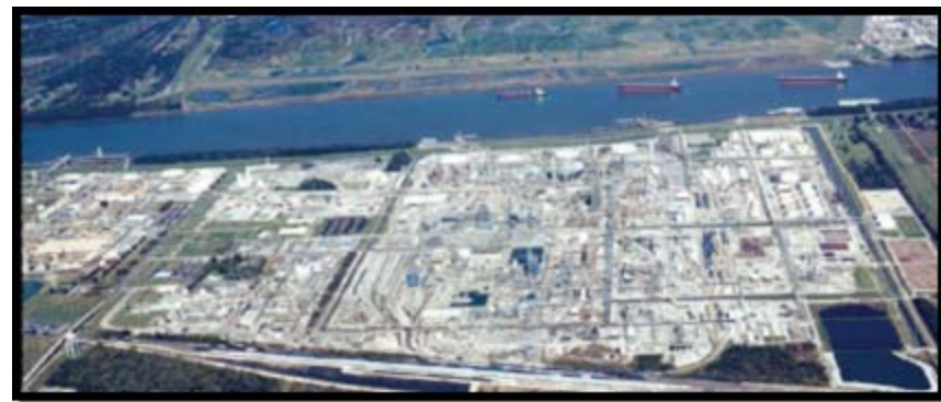
Dow Chemical's plant in Hahnville, LA
